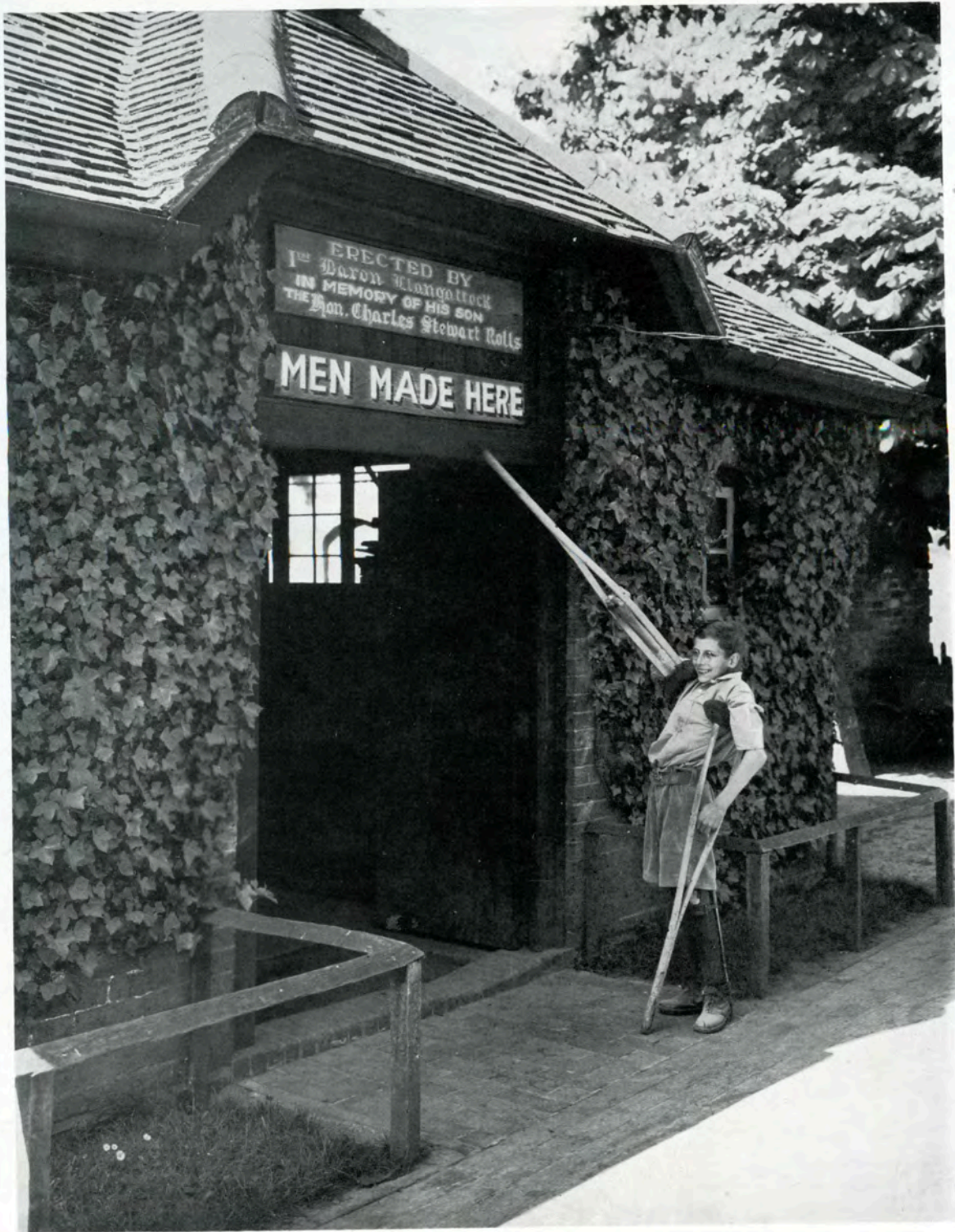
The Llangattock Carpentry Shop
