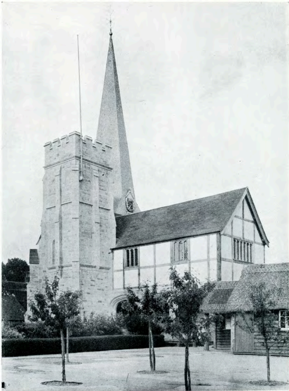
The Chapel, showing the Douty Song School and Water Tower.
